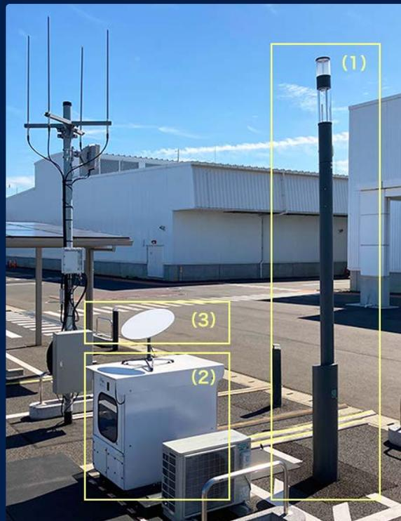
The Zella Hut outdoor data centre is an integral part of this project as it allows to store and process data at the edge, by the smart pole. Main benefits:
